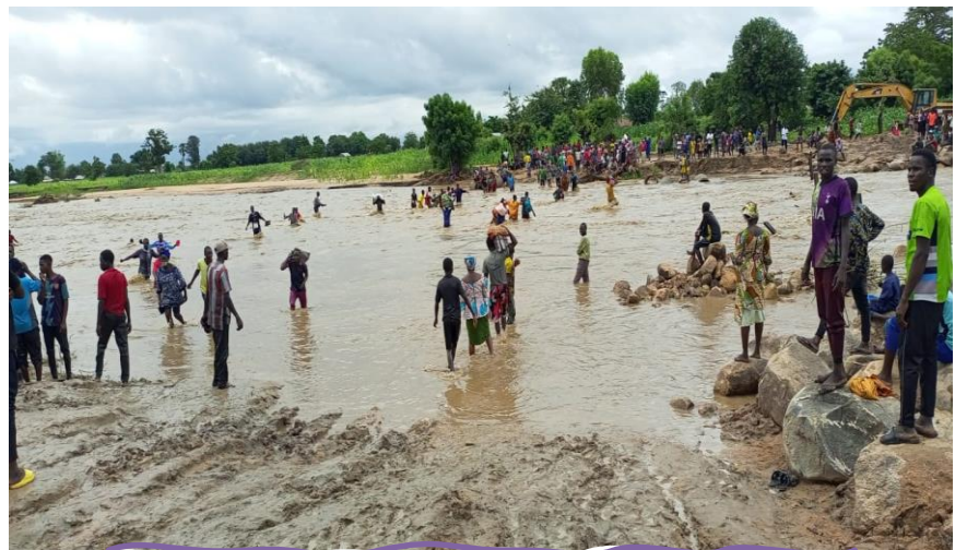
Crossing the collapsed bridge from Michika to Shuwa
